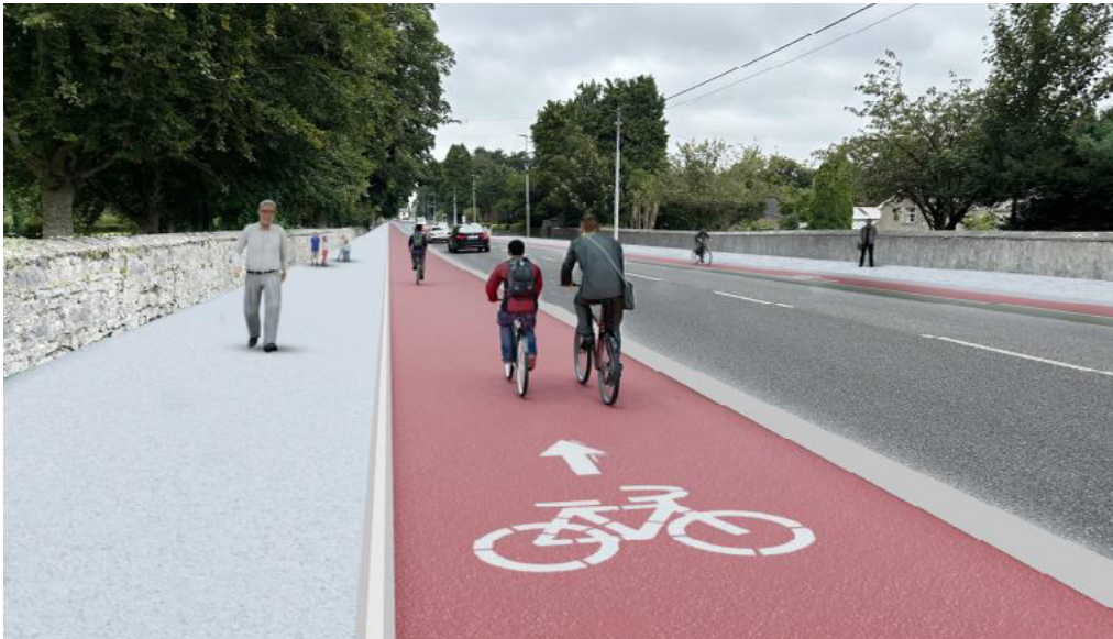
Battery Road Active Travel Scheme in Longford
