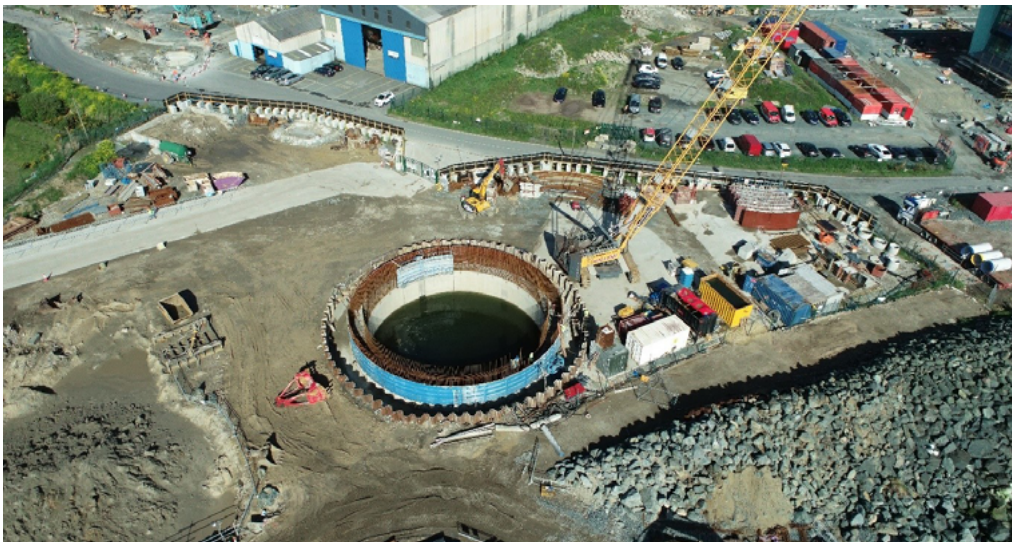
Construction of the Inlet Pumping Station
