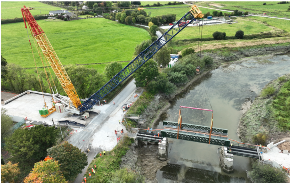
At Adare, County Limerick, the Maigue River bridge refurbishment. more details on projects across Ireland's railway network can be seen on this interactive map: https://www.irishrail.ie/en-ie/interactive-map
