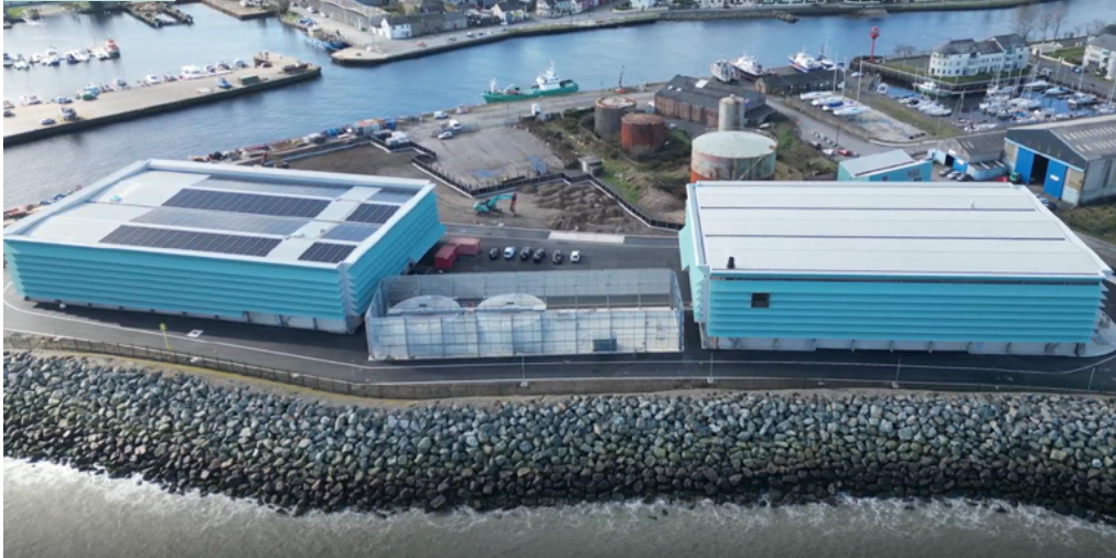
Completed Arklow Wastewater Treatment Plant Site
