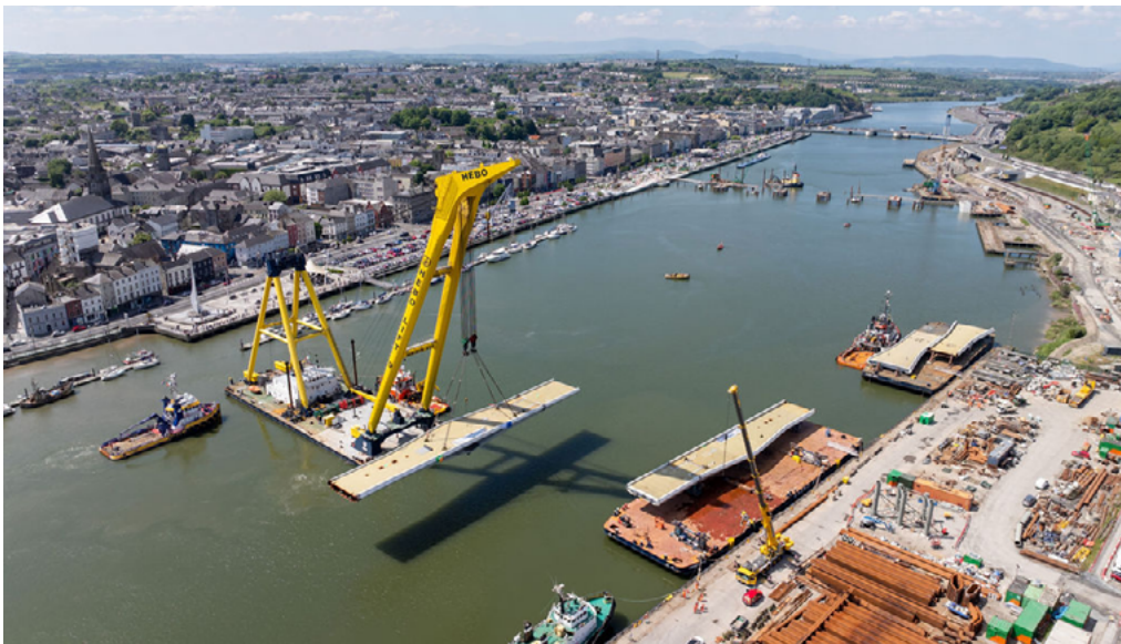
The HEBO 9 shearleg crane lifts the South Main Span into place, at Waterford's new Sustainable Transport Bridge.
