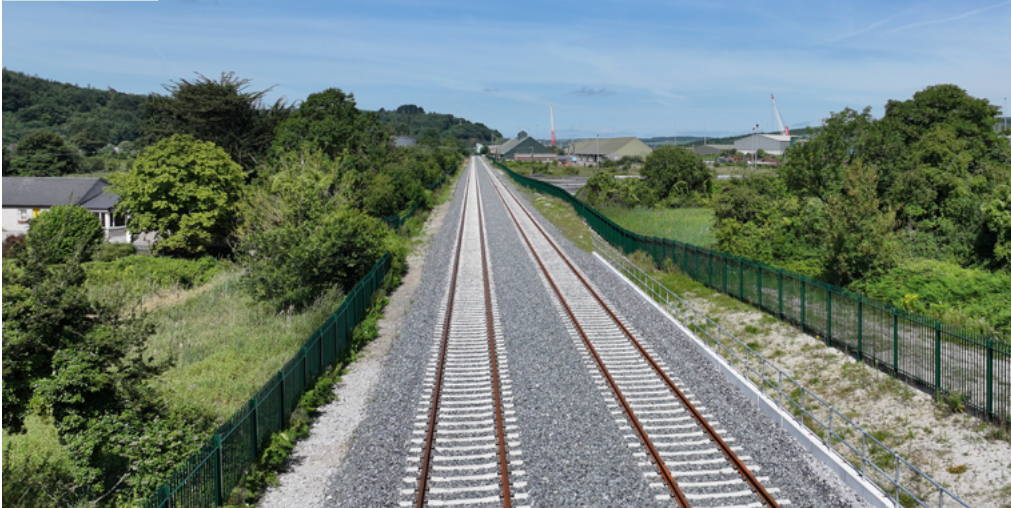
Installation of new trackbed looking towards Foynes port in county Limerick.
