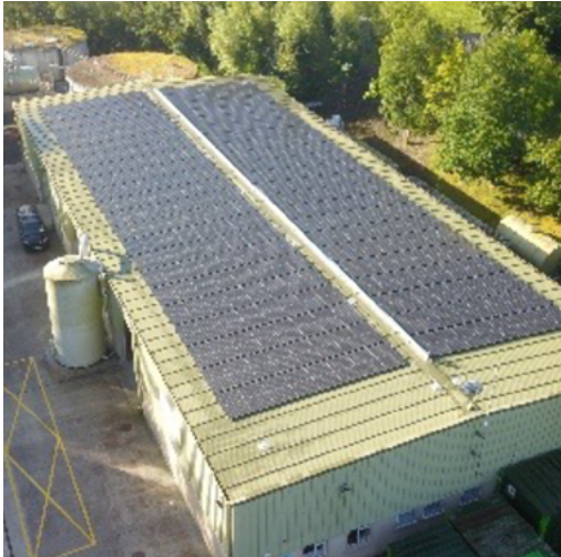
Portloman Water Treatment Plant, Mullingar, County Westmeath
