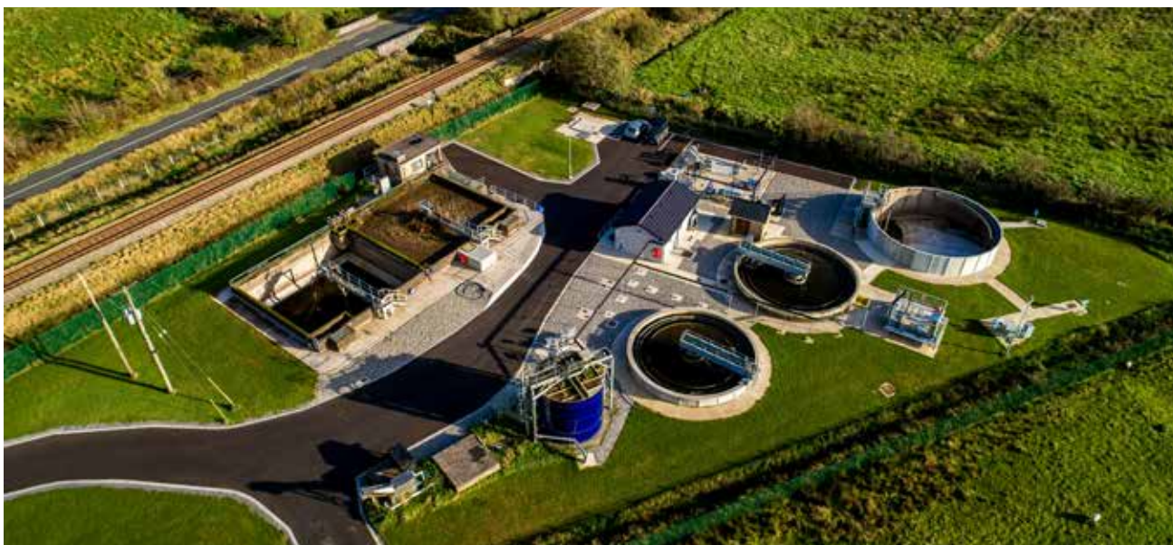
▲ Ballymote Wastewater Treatment Plant in Co. Sligo, operated by Uisce Éireann.
